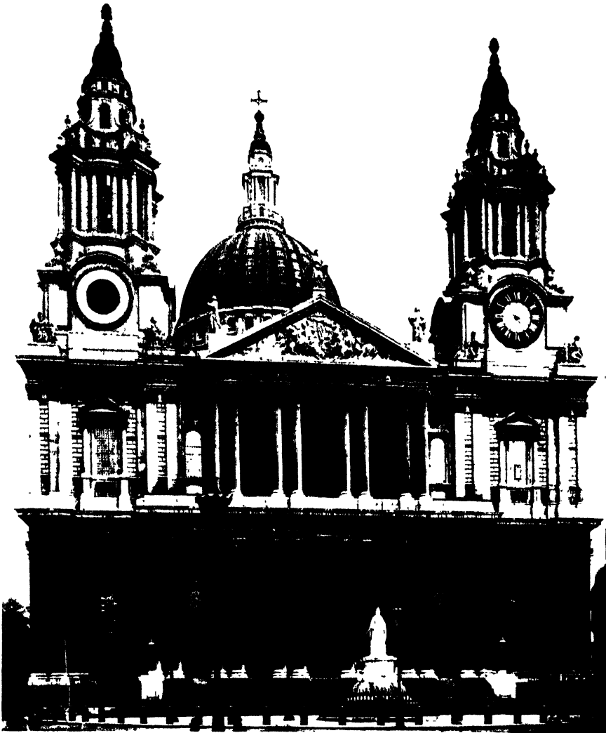
291. A seventeenth-century Cathedral: St. Paul's, London. Built by SIR CHRISTOPHER WREN from 1675 to 1710
